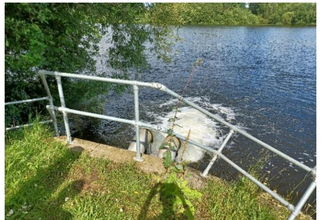
Image (right) The outflow of a small raw water transfer (credit APEM Ltd)
