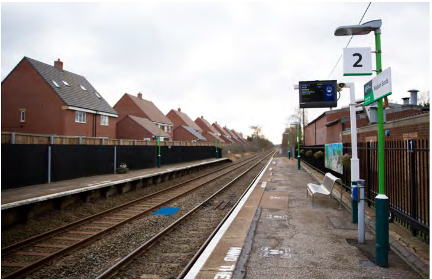
Wodburn Sands station
