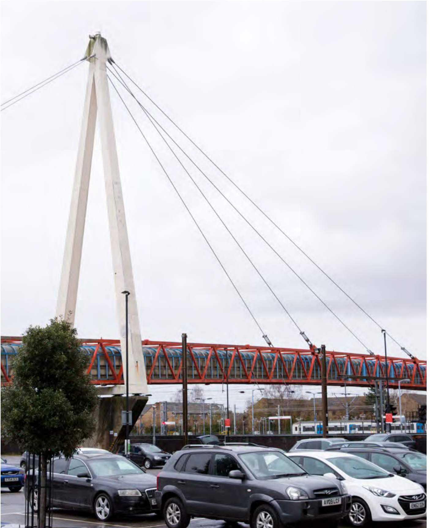
Cambridge station, footbridge
