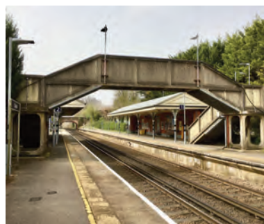
Precast concrete, Clandon
