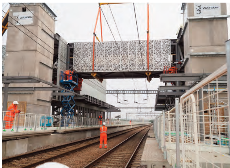
Cambridge North under construction
