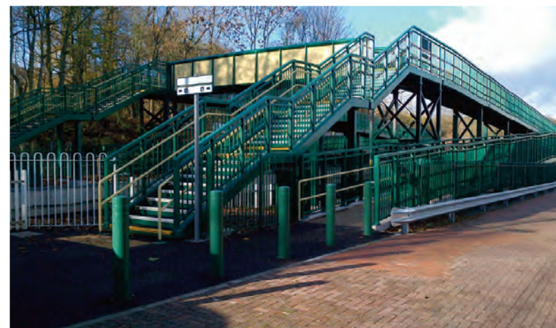
Access for All-funded footbridge with ramps, Chirk
