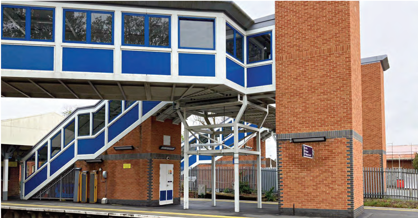
Access for All-funded footbridge, Brockenhurst
