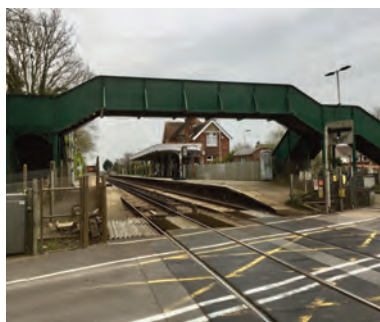
Plate girder, Bosham
