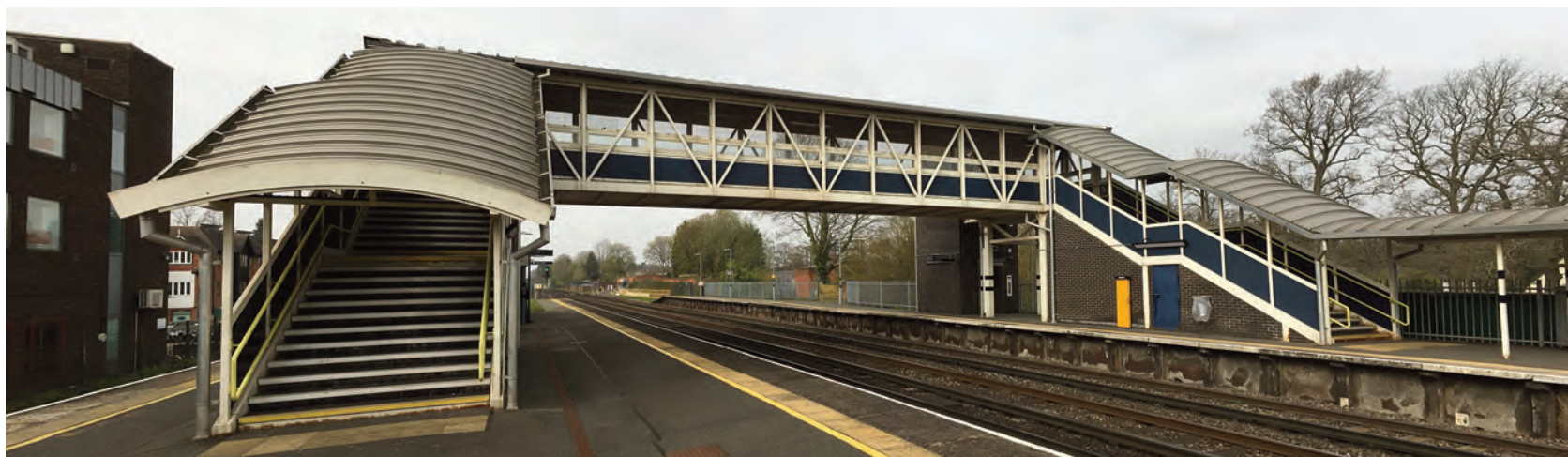
Access for All-funded footbridge, West Byfleet
