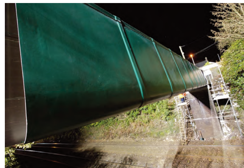
Installation of FRP bridge at St Austell
