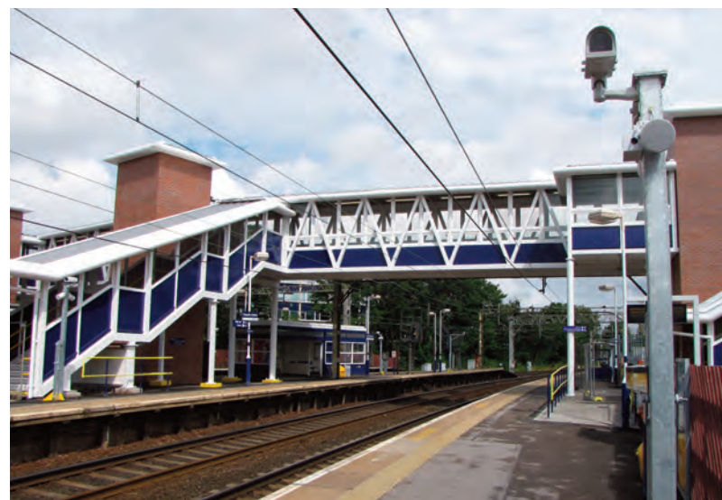
Access for All-funded footbridge, Cheadle Hulme
