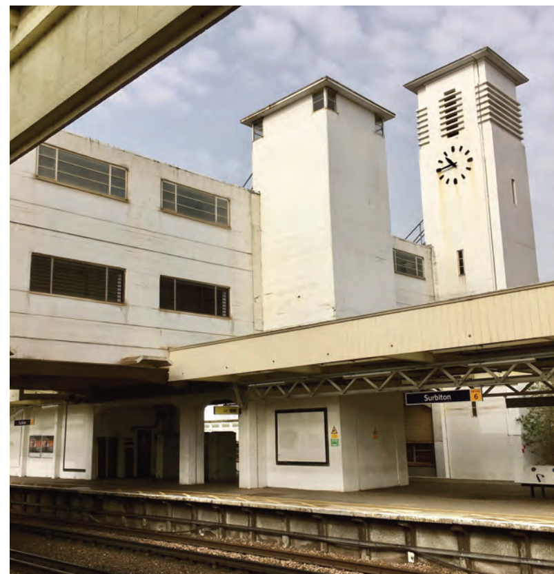
Double-deck footbridge, Surbiton
