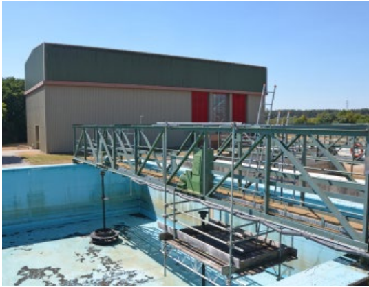
Figure 6 – Part of the ALES facility
