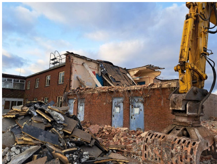
Figure 9 – Demolition of ancillary building A44 at the Winfrith Site
