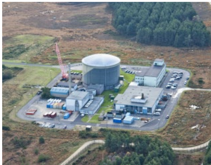
Figure 5 – The Dragon reactor with ancillary buildings
