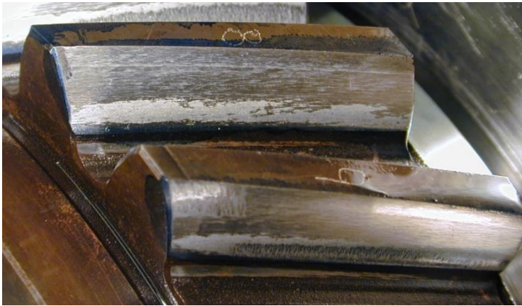
Figure 7. Gear micro-pitting (grey staining) contact fatigue damage.
