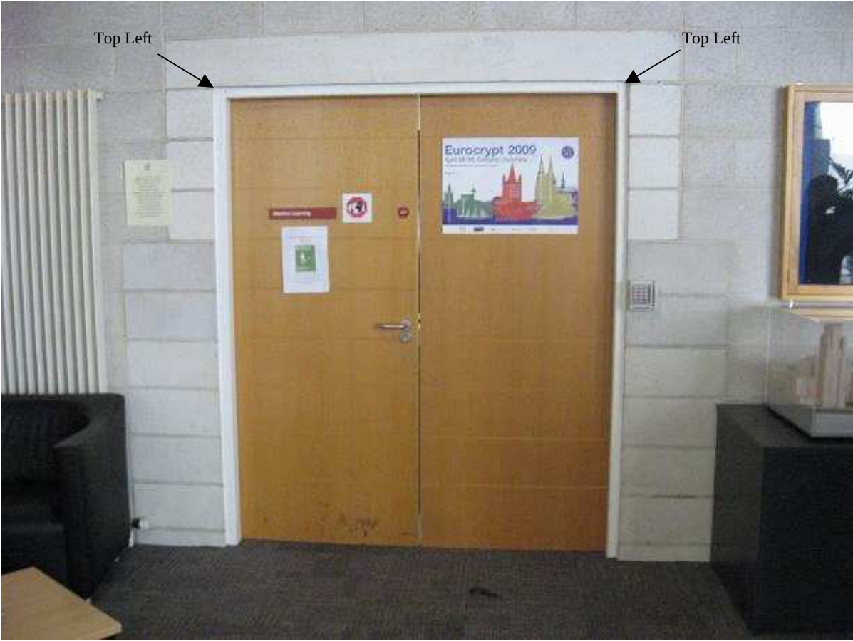
Figure 32 Features on Room 2.01 door surround.
