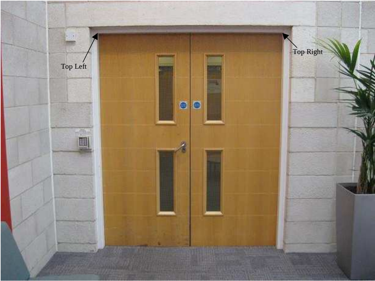
Figure 29 Features on the 'Set Squared' Door. The top outer corners of the frame.
