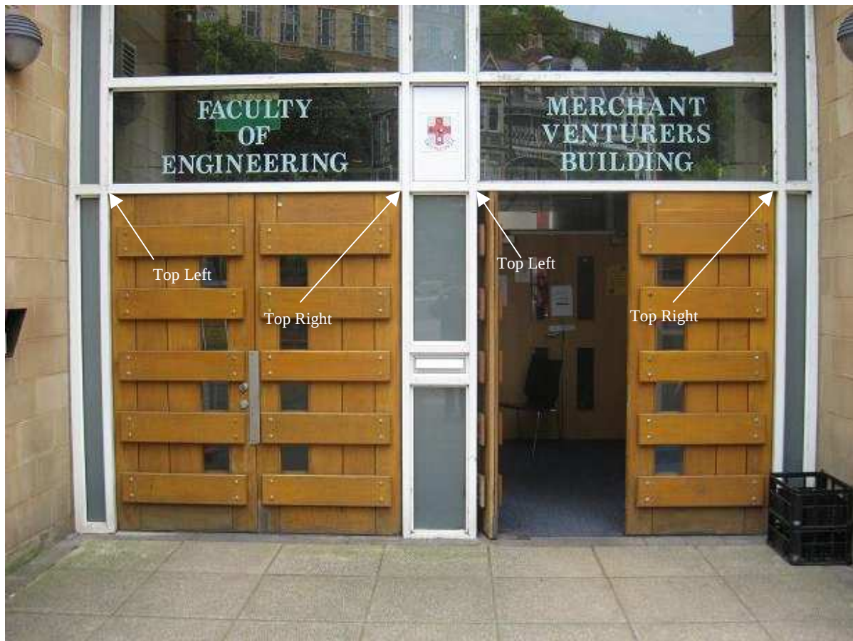
Figure 30 Feature round the Main entrance doors. The top corners of the left and right doorframes.
