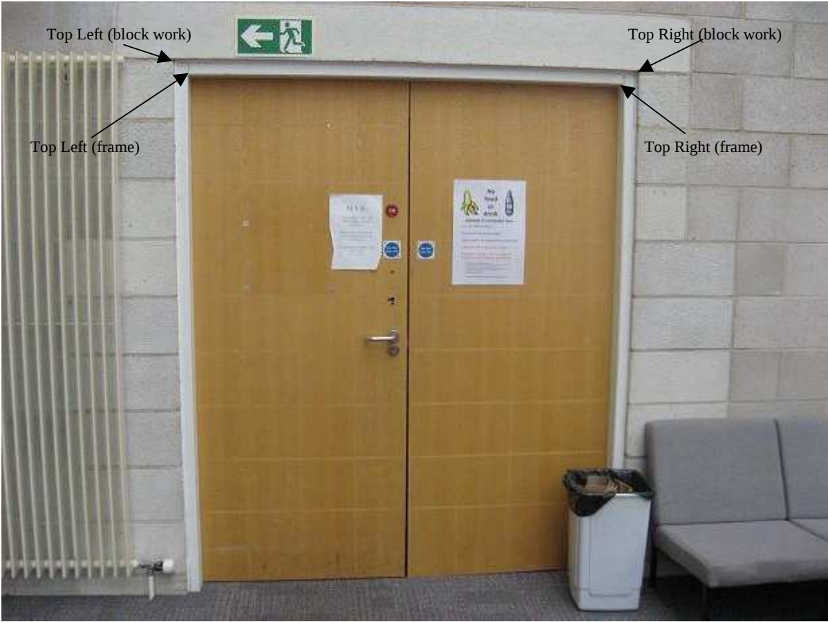
Figure 27 Feature on Room 2.16 door.
