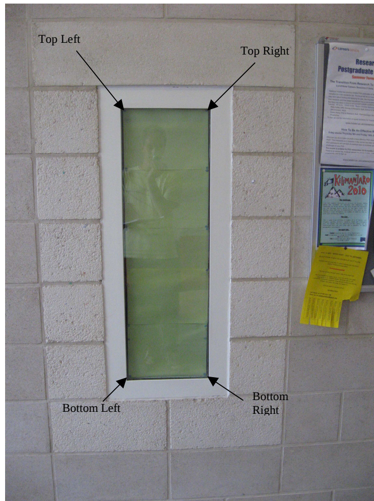
Figure 22 Features on the False Window on the lower floor. Corners of the glass pane.
