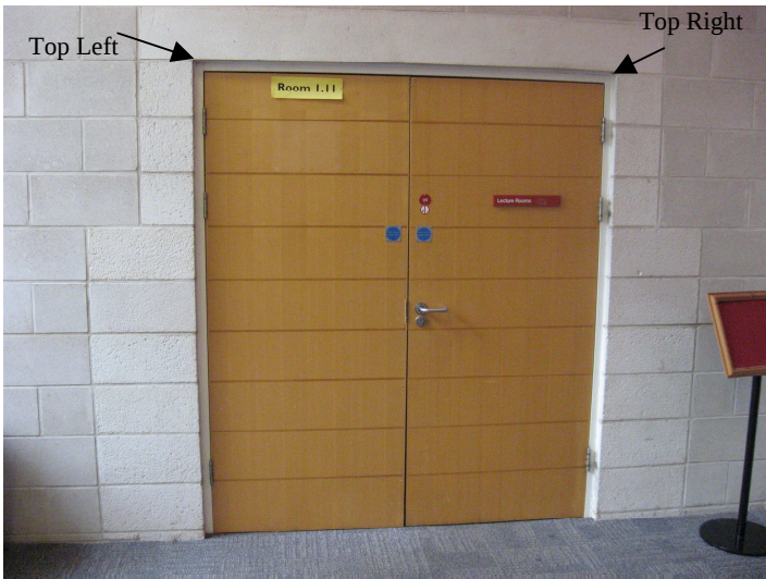
Figure 20 Features on Room 1.11 door. Outside corners of block work.
