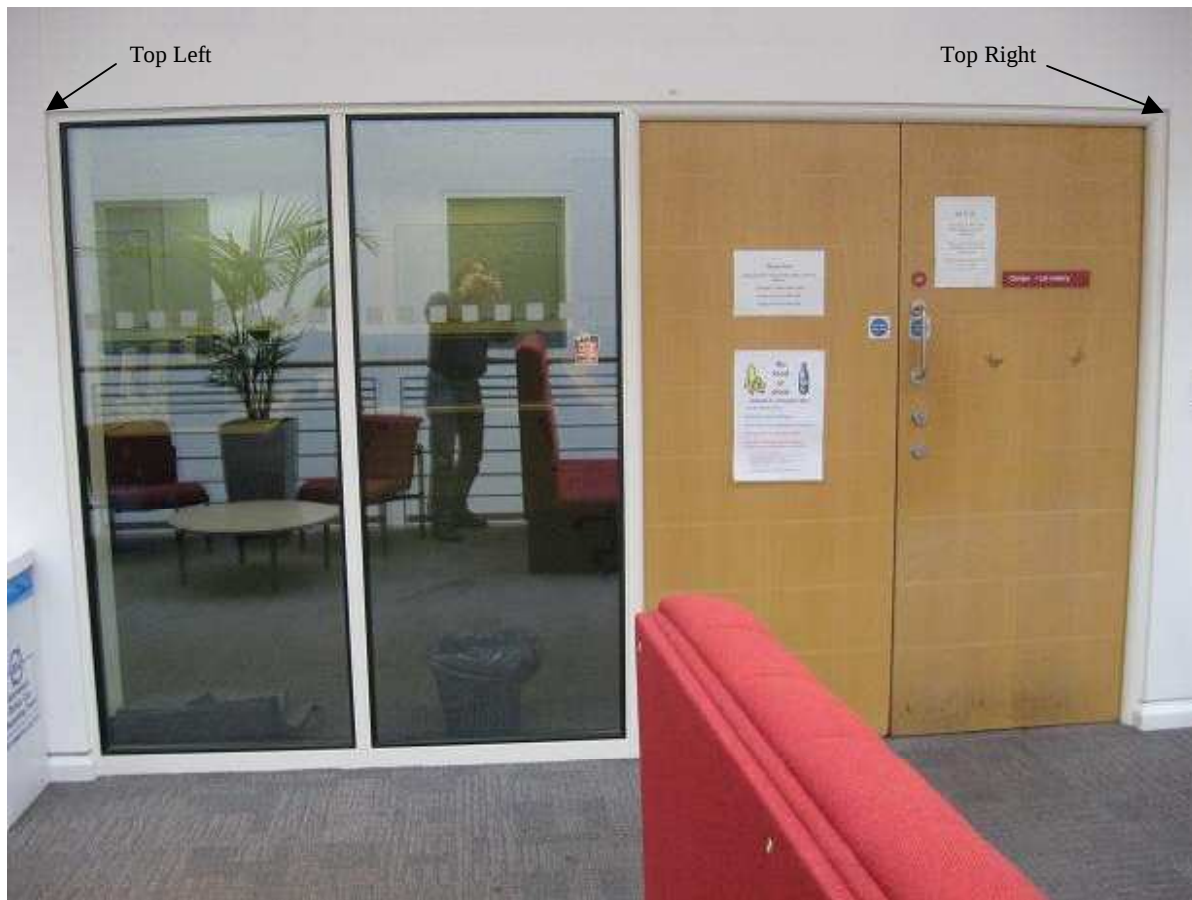
Figure 26 Feature on Room 2.11 Door/Window surround.
