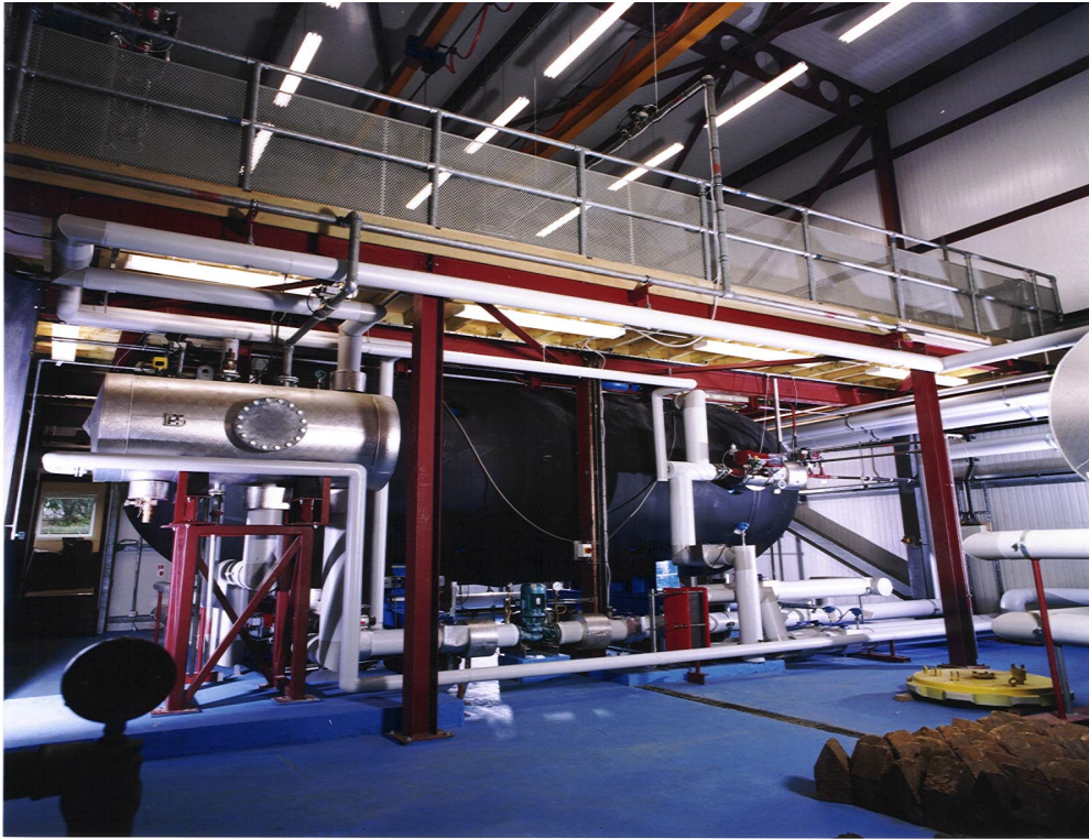
Figure 1.5: Plant room area.
