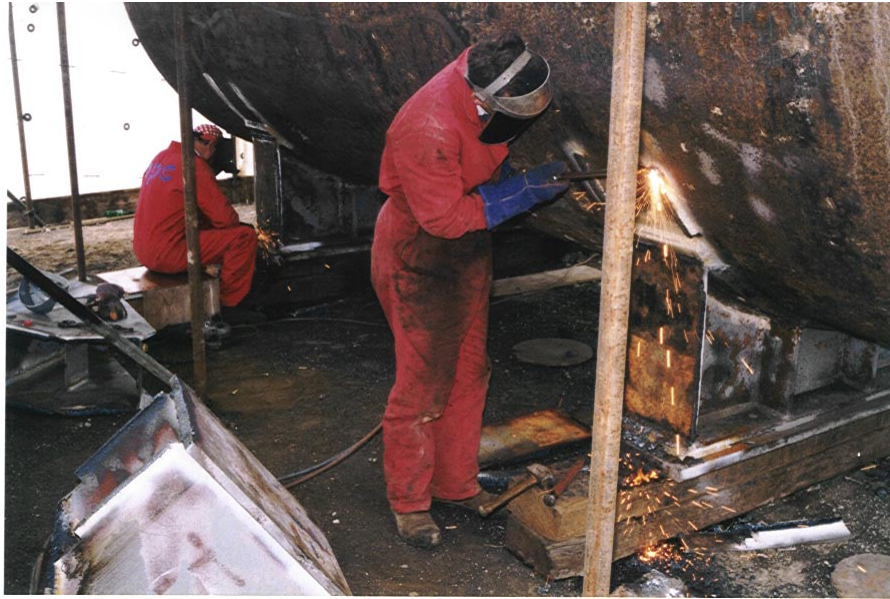
Figure 1.3: Outriggers being replaced.
