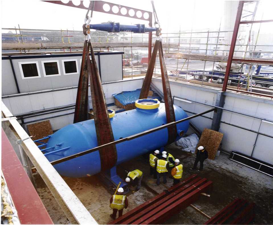
Figure 1.4: Vessel being positioned in new building on the NPL site.
