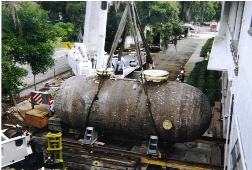
Figure 1.1: Vessel being prepared for lifting.
