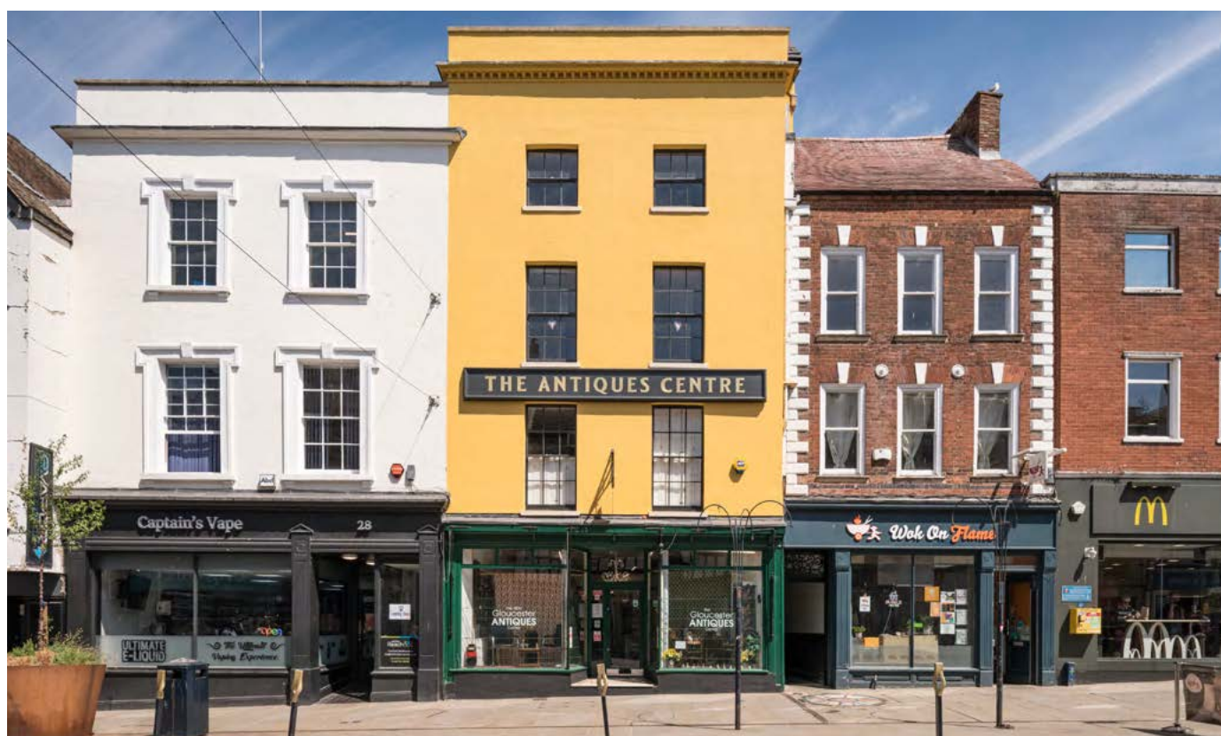
26 Westgate (Old Judges House), Gloucester, the largest timber-framed townhouse in England was saved.
