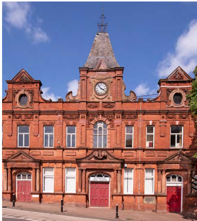
Netherton Public Hall and Free Library in Dudley, West Midlands, now known as Netherton Arts Centre, was newly listed at Grade II in 2025.
