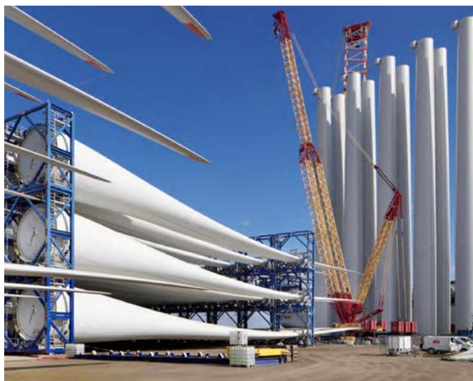
The turbine installation yard for the Dogger Bank Wind Farm at Able Seaton Port, County Durham.
