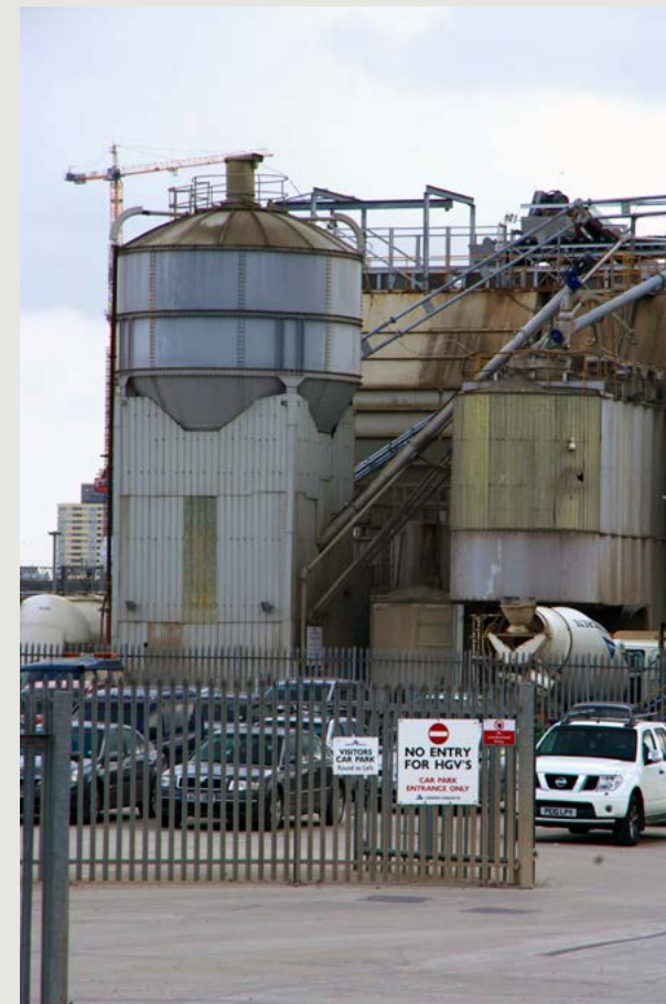
Concrete batching plant, Wick Lane
