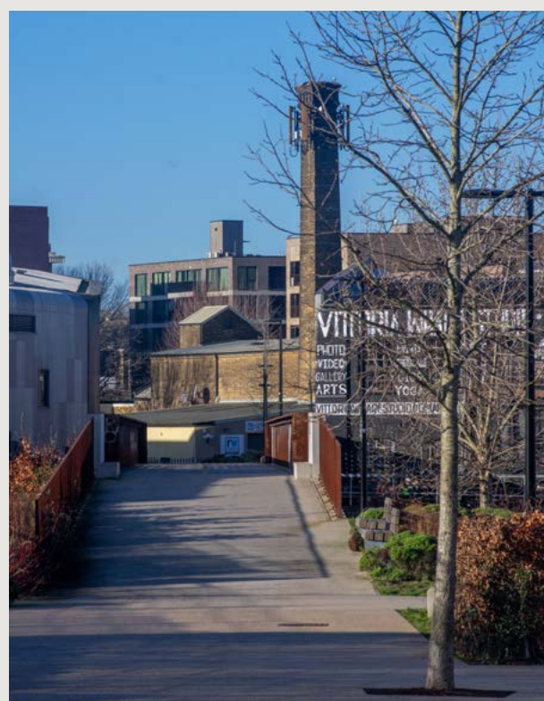
New pedestrian and cycle bridge to Stour Road
