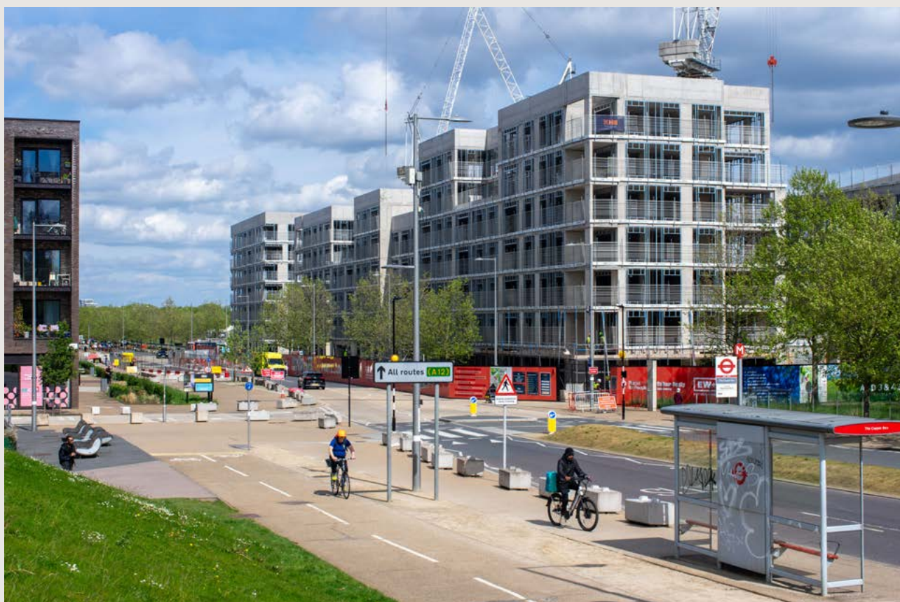
Legacy Community Scheme, Phase 2 East Wick, 210 homes under construction
