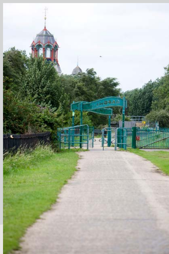
Abbey Mills Pumping Station (Credit: David Poultney)
