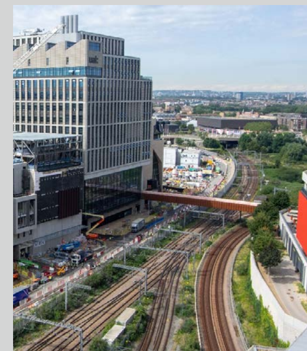
Carpenters Land Bridge, connecting Stratford Cross and East Bank
