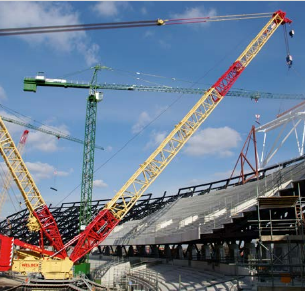
Above: construction of the London Stadium
