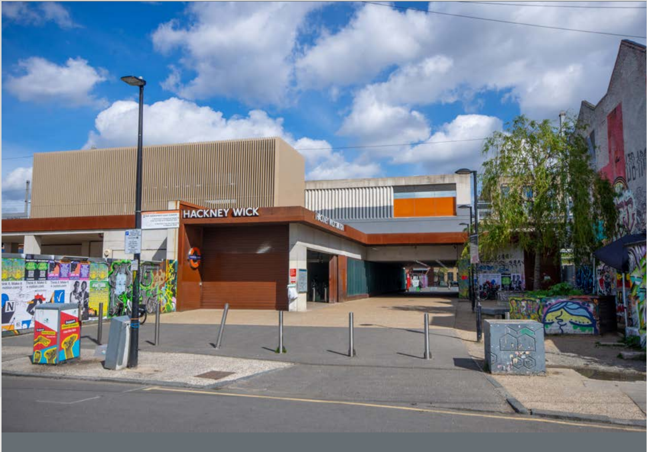
Hackney Wick Overground Station
