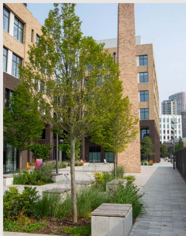
Reinstated chimney, Sugar House Island
