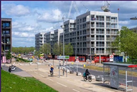
East Wick Phase 2 homes under construction, along Waterden Road
