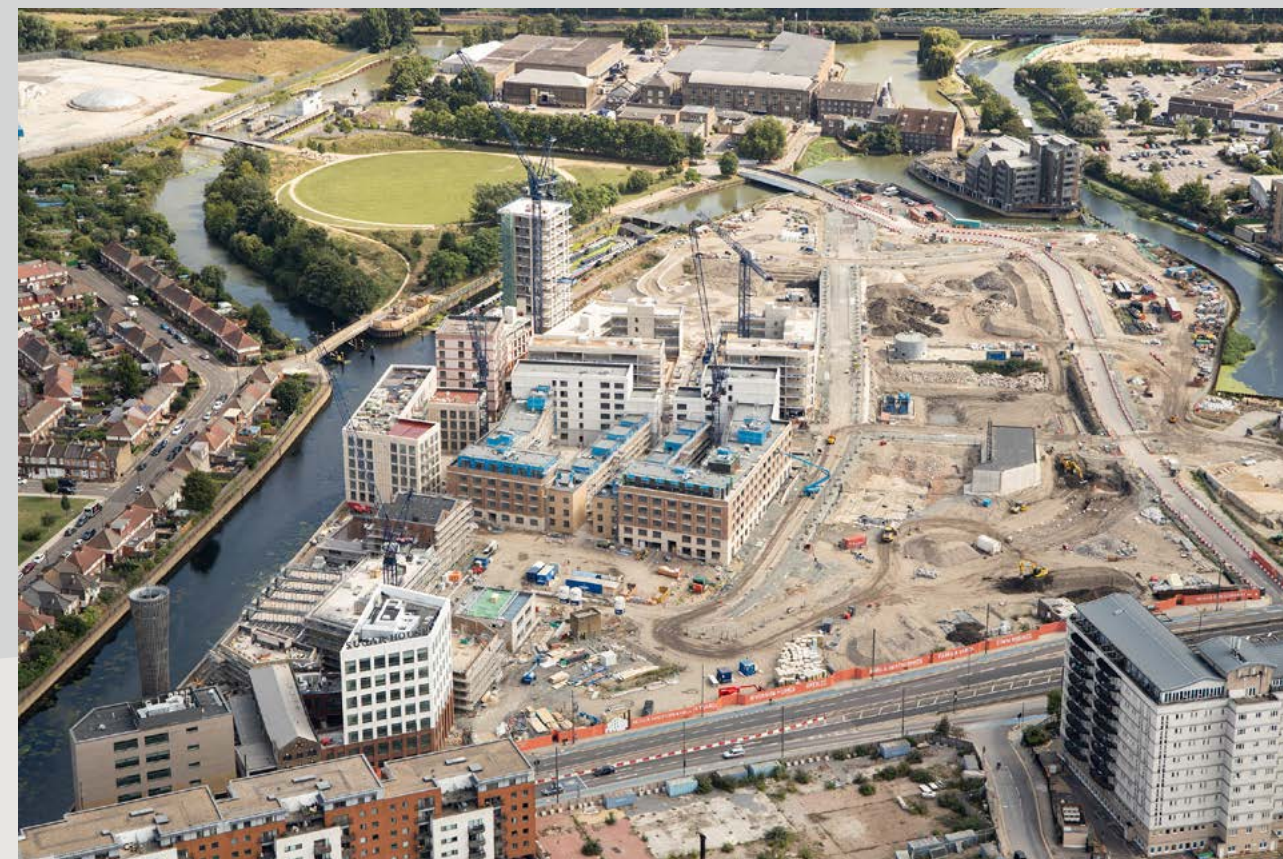
Sugar House Island first phases out of 1,100 homes under construction in 2021.
