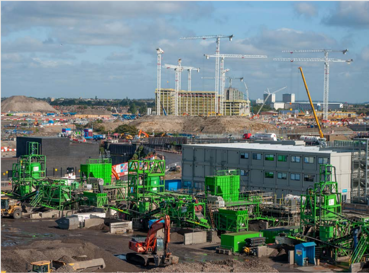
Below: remediation of the Park, 2009
