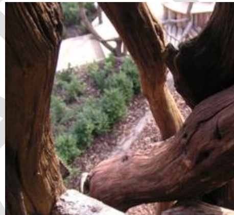
Entrapments in a downwards direction
