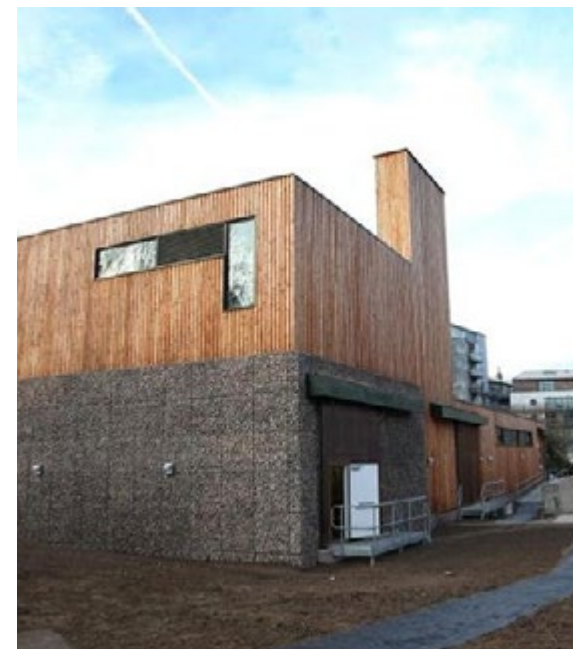
Old Ford Water Recycling Plant.
