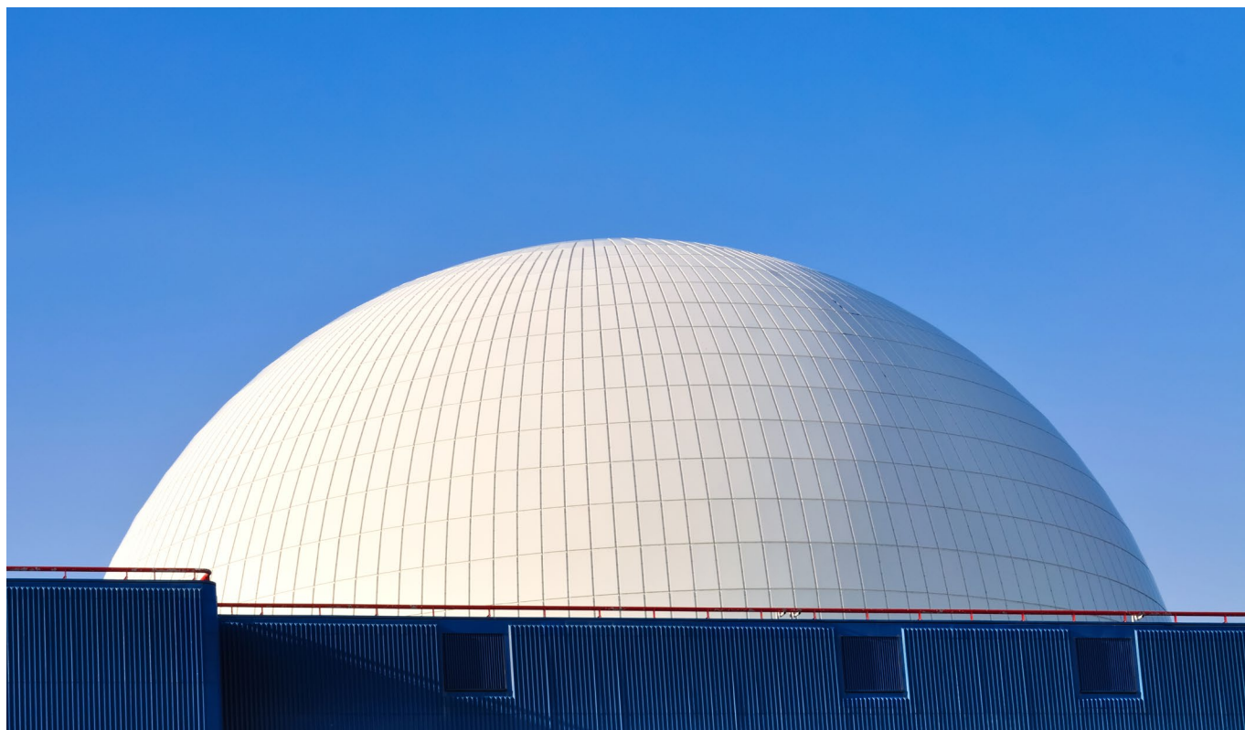
The white reactor dome at Sizewell B nuclear power station in Suffolk, UK
