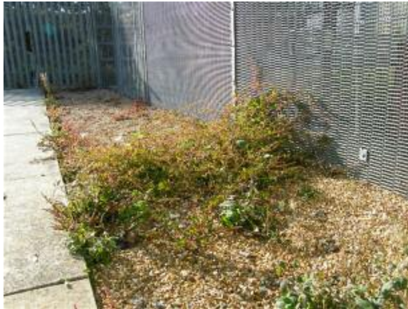
Figure 4: Movement of vegetation such as this against the fence can cause false alarms for barrier-mounted PIDS
