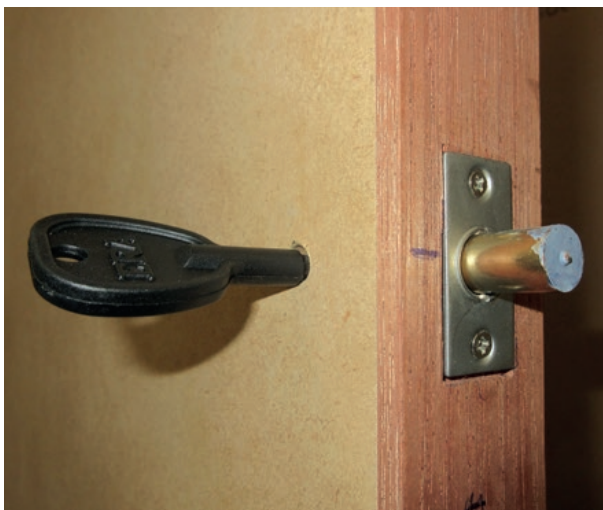
Figure 7: Low-cost key-operated door bolt retrofitted to a hardwood timber door
