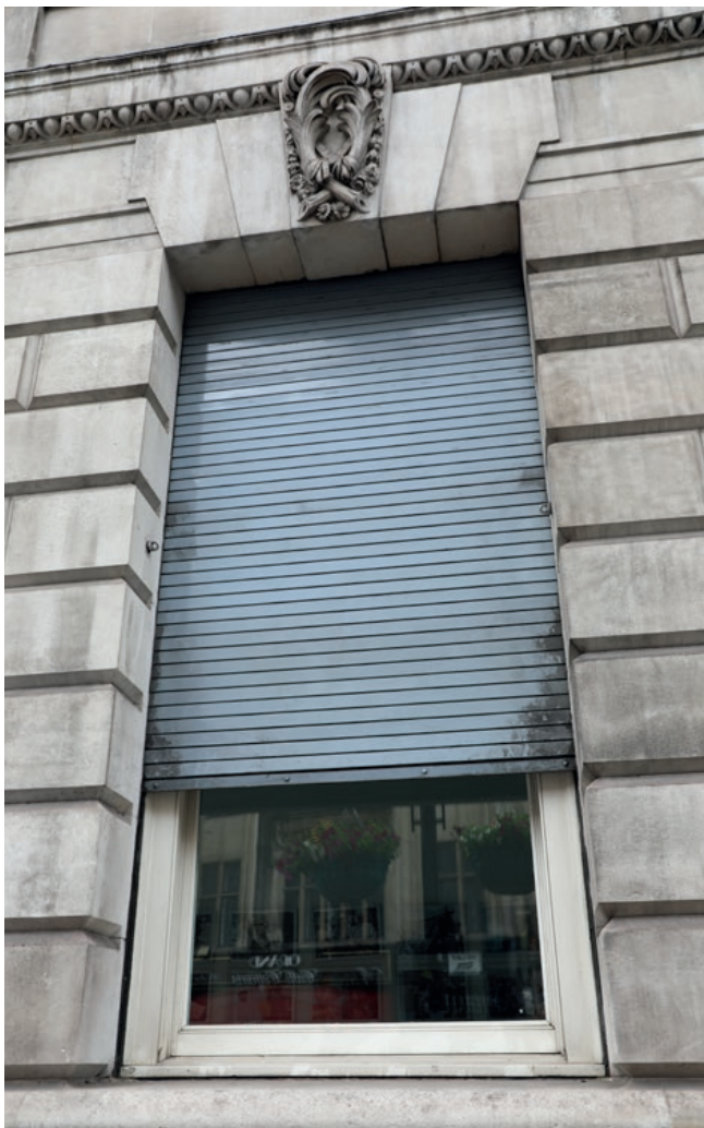
Figure 15: Roller shutter covering a window
