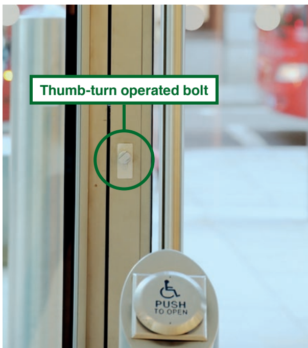
Figure 8: Thumb-turn operated secondary door bolt fitted to an external door constructed with framed glazing
